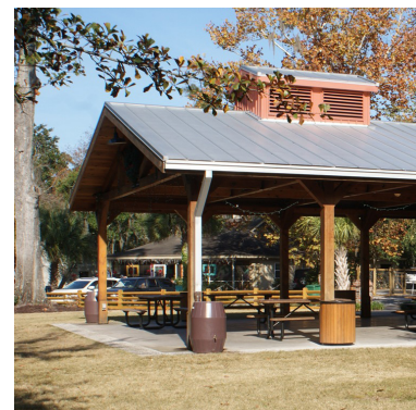
Figure 23 Pavilion(Kenneth Scott Builders)
