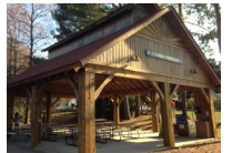
Post and beam picnic pavilion
