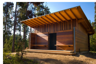
Figure 24 Composting toilet examples: TOP: Grand Teton NP (courtesy of Clivus Multrum)
