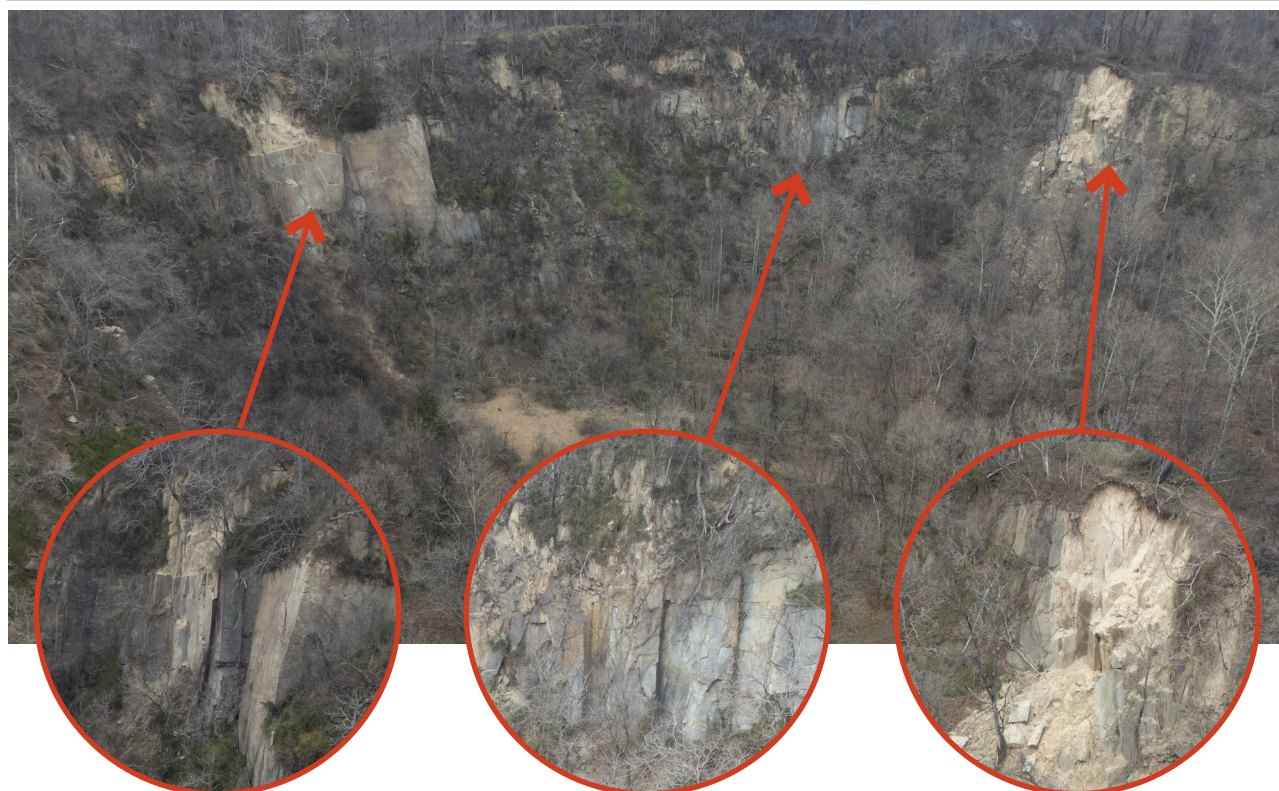
A. Hard granite rock faces (south facing quarry wall)
