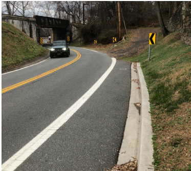
View from North Main toward Mill Street entrance
