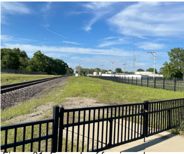
Figure 31 Example of fencing along freight rail lines designed to deter inadvertent crossings
