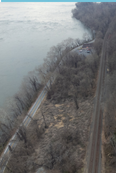
Aerial view looking north towards VFW
